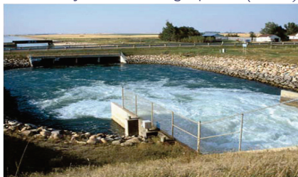
Tehama Colusa canal system (2007)
